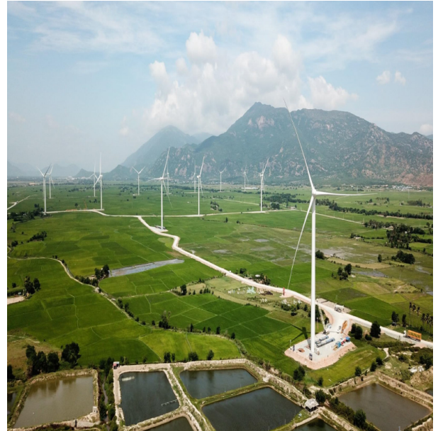
The above picture is of the Dam Nai wind project financed by Armstrong Asset Management in Vietnam which was Vietnam's first foreign-owned wind project
